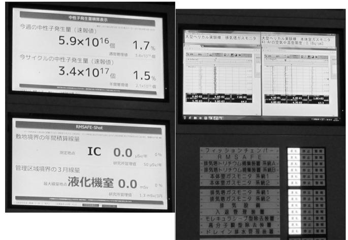
Figure 5: Three radiation monitoring displays and the interlock status indicator (right bottom): Top three screens usually show weekly and yearly neutron yield, plasma derived yearly and three-month cumulative doses (Sv), and gas radioactivity concentration (Bq/cm<sup>3</sup>) at the exhaust tower and the torus hall, respectively.
