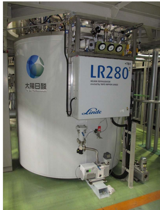
Fig. 2. Photograph of the variable-temperature helium refrigerator/liquefier.
