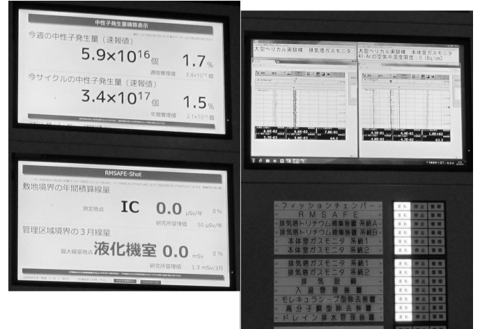
Figure 5: Three radiation monitoring displays and the interlock status indicator (right bottom): Top three screens usually show weekly and yearly neutron yield, plasma derived yearly and three-month cumulative doses (Sv), and gas radioactivity concentration ( \text{Bq}/\text{cm}^3 ) at the exhaust tower and the torus hall, respectively.
