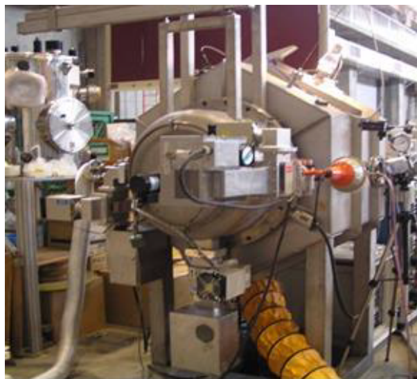
Fig. 1 Test furnace of 2.45 GHz magnetron system.
