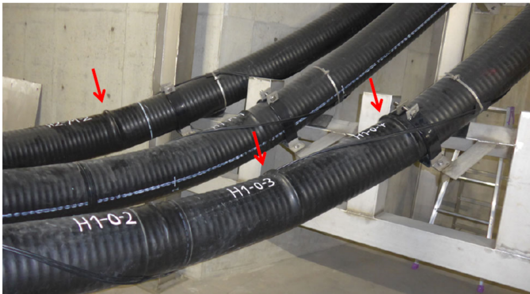
Figure 7. Photograph of three kinked portions of the bus lines for the helical coils.
