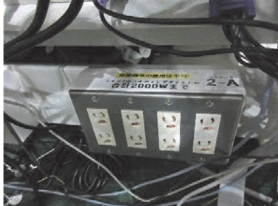
Fig. 12 Outlets for data acquisition system power supplies in the Thomson scattering system.
