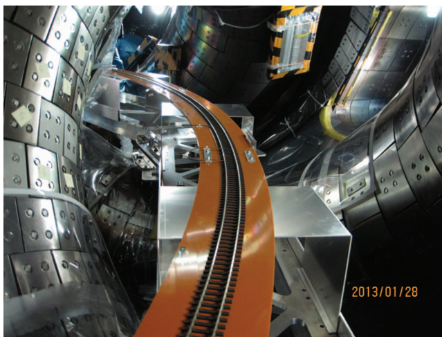
FIG. 6. Test installation of track inside the LHD vacuum vessel that will be used for in situ NFM calibration.
